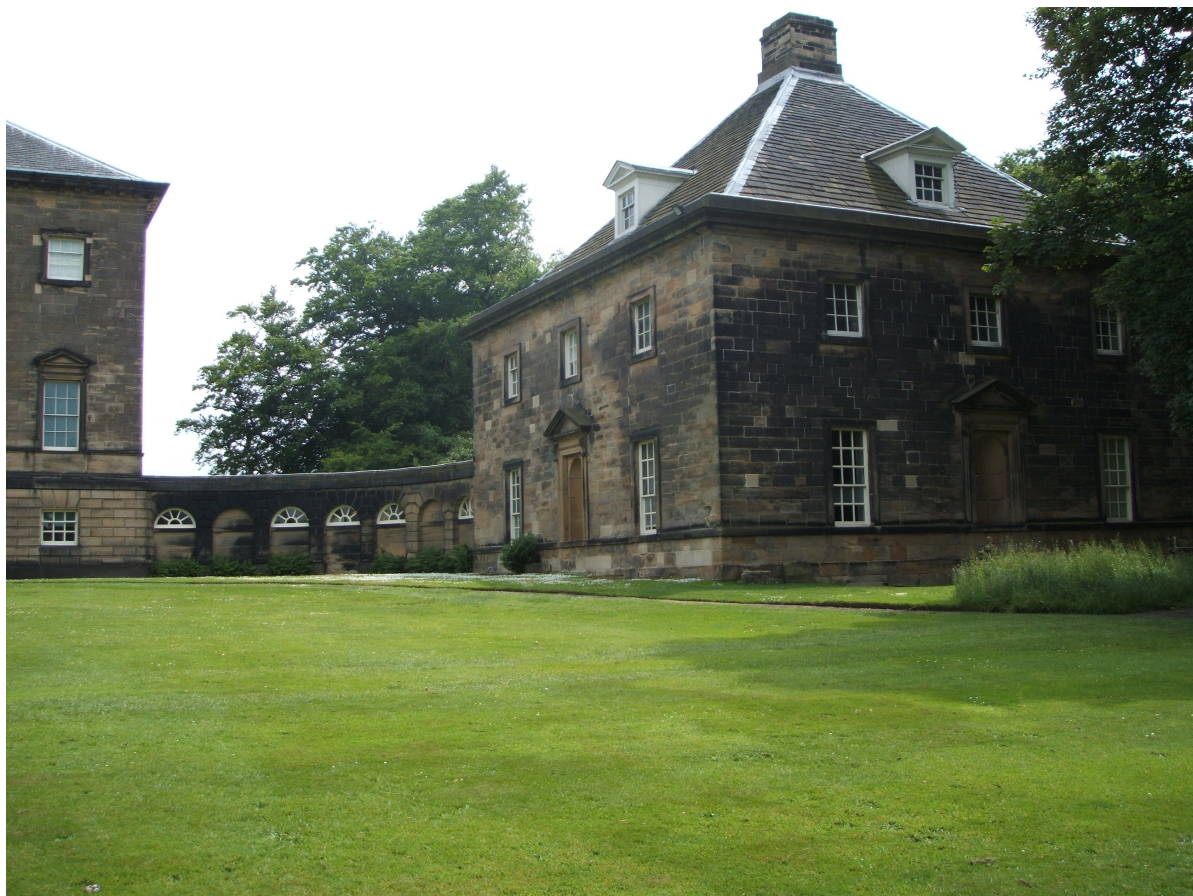
Fig. 25. Nostell Priory , West Yorkshire: west front of the Kitchen pavilion and link (author's photograph).
