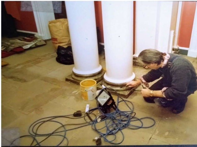
WORKING ON THE HALL PILLARS
